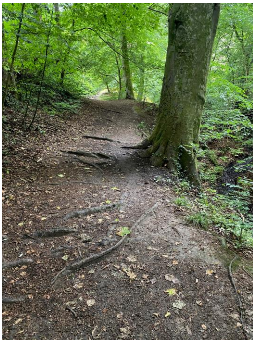
Photo of path to be formalised with compacted aggregate and edging boards on the right to regulate levels. Tree roots to be retained and built over.
